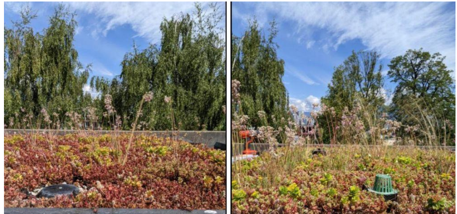
Comparison of the green roof (left) and connected blue-green roof (right) on July 17, 2021 during the 2021 heat wave
