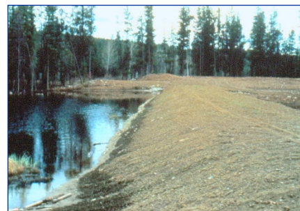
Figure 5.1 A Sample Dam
