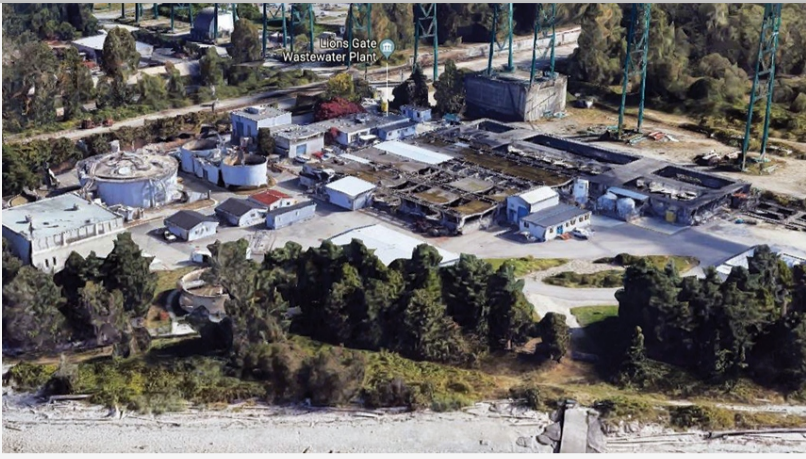
The 58-year-old Lions Gate Sewage Treatment Plant on the shores of Burrard Inlet, a primary treatment plant, is set to be replaced. image Google Maps
