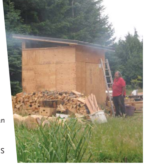
The smokehouse, designed and built with leadership from First Nations elders in UBC Farm's Aboriginal Community Kitchen Garden, provides an integrated learning experience for second-year Civil Engineering students.
