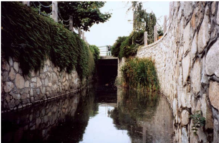
Confining and channelizing of Bowker Creek
