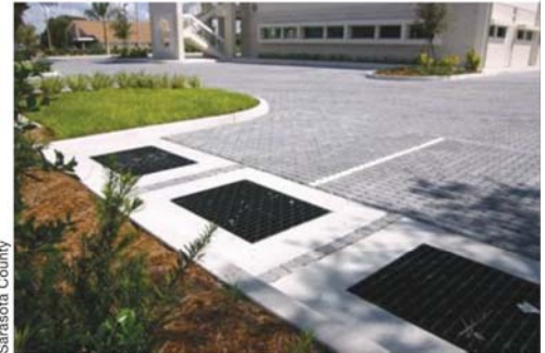
This LEED office building features all-pervious parking.
