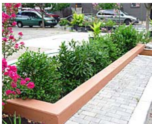
Philadelphia Water Department A stormwater planter at Columbus Square in Philadelphia.
