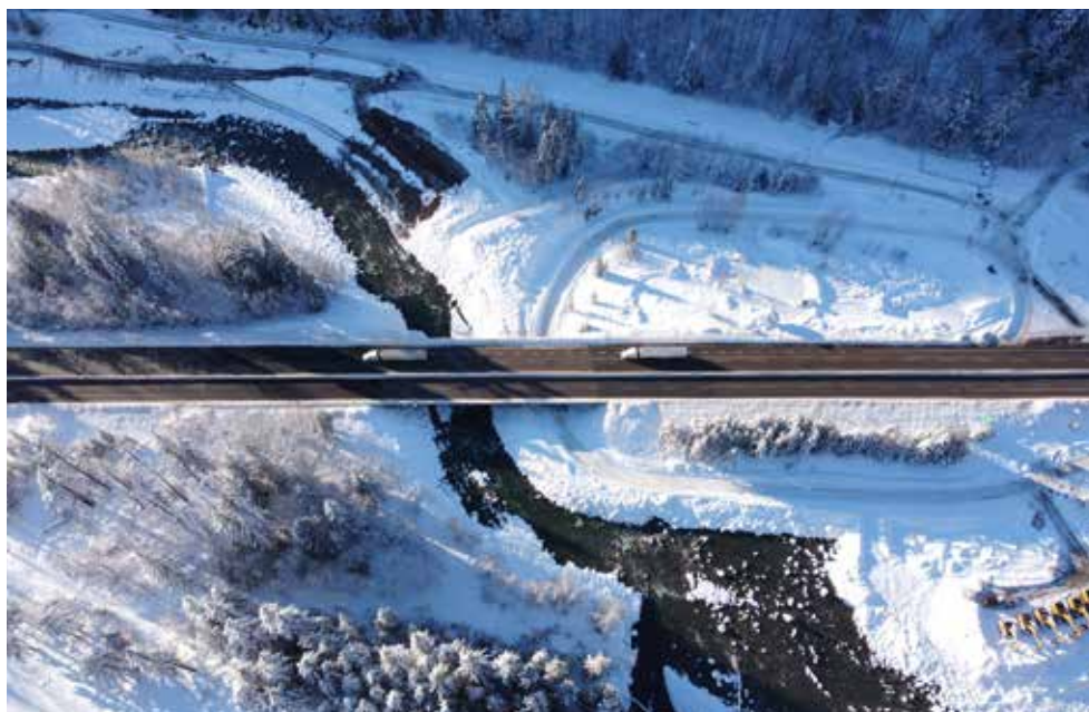
■ Top: Westridge Marine Terminal. Middle: YVR North Runway Program. Bottom: B.C. Highway Reinstatement Program
