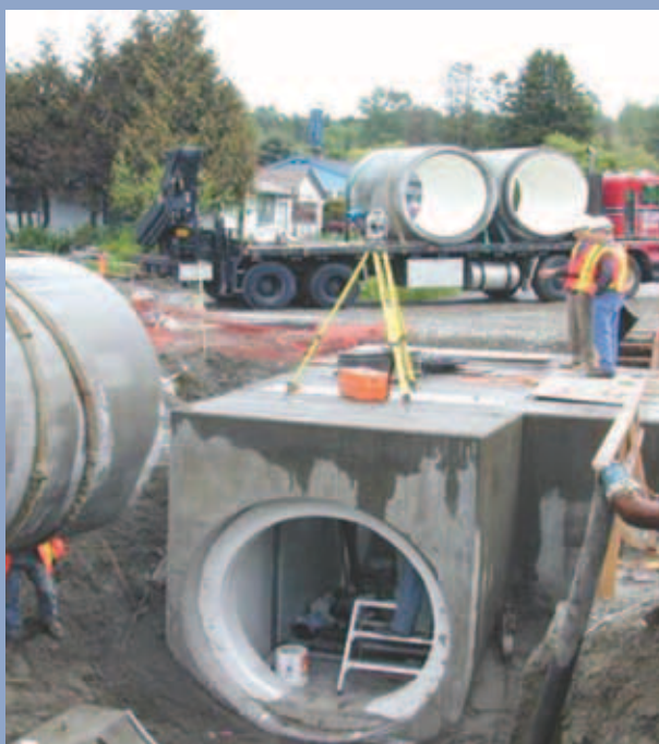
Installing Metro Vancouver trunk sewers, South Surrey.
