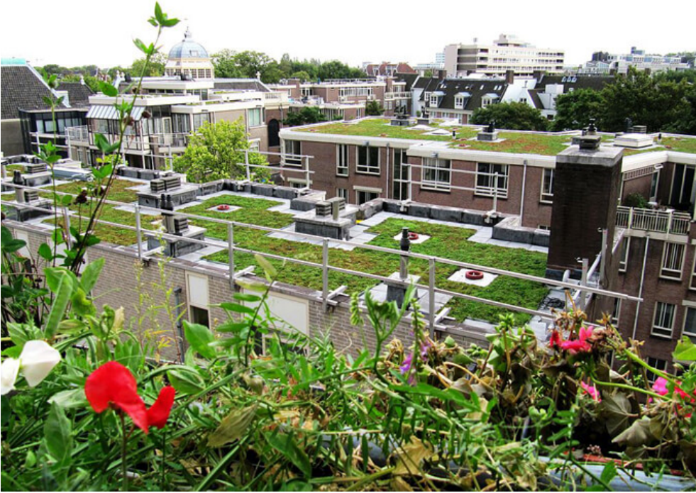
Green roofs in Amsterdam. By Picasdre (Own work) [CC BY-SA 3.0] or GFDL, via Wikimedia Commons. Typically, with heavy rainfall, water is
