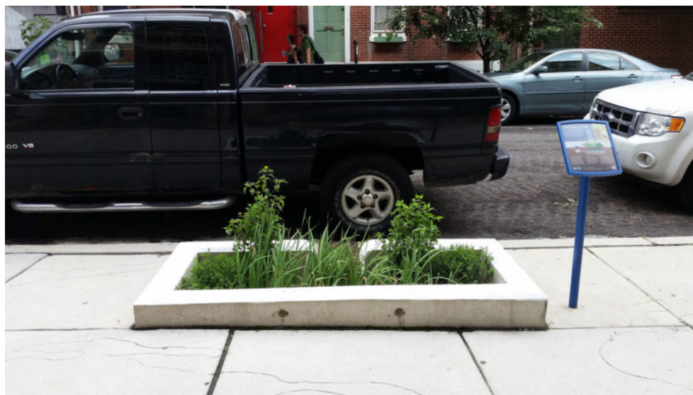
New planters on Philadelphia sidewalks capture runoff from the streets. PHILADELPHIA WATER DEPARTMENT
