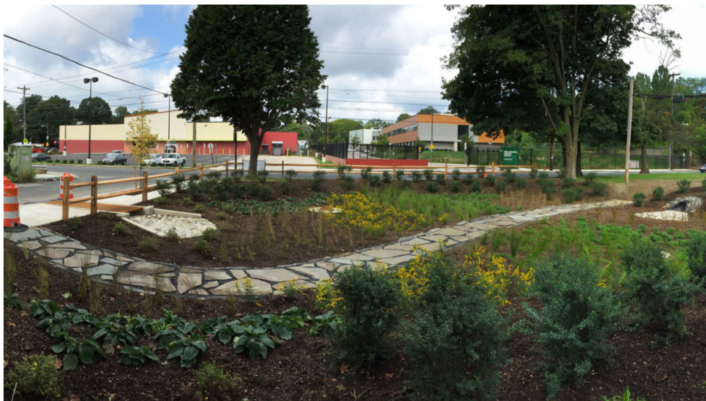
A rain garden manages stormwater runoff in Philadelphia's Germantown section. PHILADELPHIA WATER DEPARTMENT
